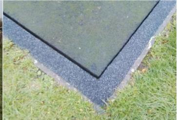
**Finding:** There are gaps opening between the surfacing and **Action:** Monitor for any further deterioration and repair as the edging surround or between the joints in the surfacing required
