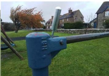
Finding: There is/are finger entrapment/s in the framework Action: Monitor - No remedial work recommended and the item fails to meet the requirements of BS EN 1176 Part 1 4.2.7.6 Entrapment of fingers
