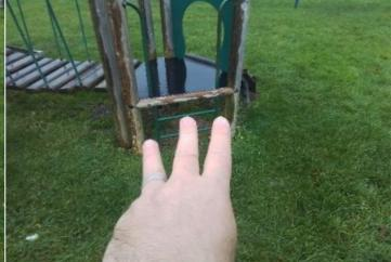
**Finding:** There are areas or parts of the posts x6 on the structure that have rotted with evidence of rot in the remaining posts
