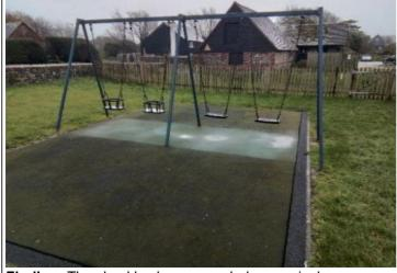
Finding: The shackles have corroded excessively
