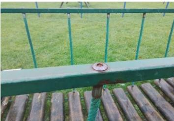
**Finding:** A number of rope fixing(s) have worked loose
