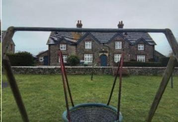
**Finding:** Swings of this design should have a secondary safety mechanism fitted to prevent collapse of the seat in the regularly event of a joint failure to comply with BS EN 1176 Part 2, however this swing was installed prior to the standards being updated in 2018 and the manufacturer has confirmed
